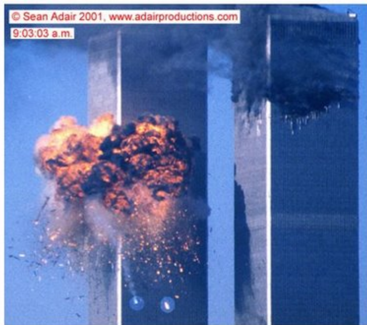
Figure 7-5. An image of the towers recorded from the north northeast is shown. The photograph was taken 4.3 s after the aircraft impact on WTC 2. Highlighted areas show two large pieces of aircraft debris that passed through the building and landed in the vicinity of the Church and Murray Streets intersection.
